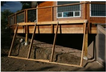
Here is the frame with 1/2'' exterior grade plywood attached to the back:
