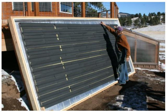
Note the slope of the grid to provide for completely draining the grid. I filled in the rest of the outside perimeter of the grid with mineral wool insulation.
