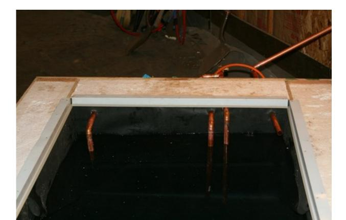
I then put holes thru the SIPs and EPDM below the top surface of the tank. This allows the tank top to go on and create a good seal. Also, notice the tube on the far right is the return tube coming from the top of the collector; it is **above** the water line.
