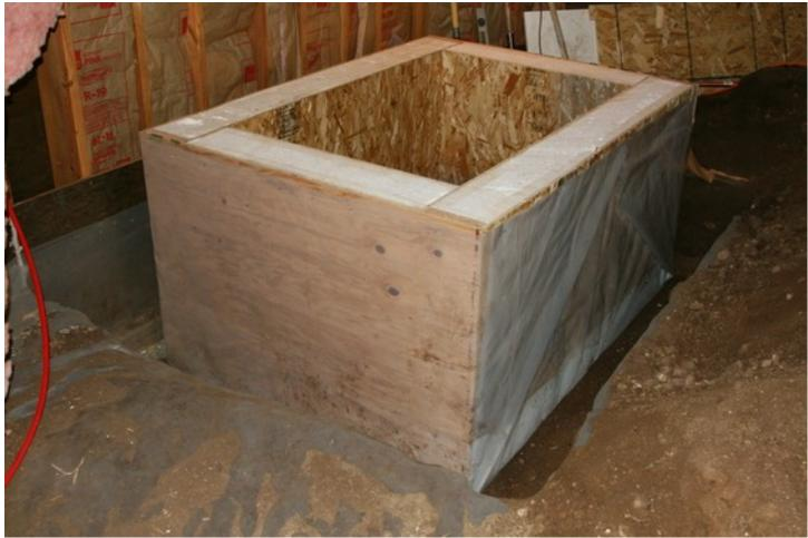
I lined the tank with EPDM. Then I put a metal channel around the top. Here is a picture showing this:
