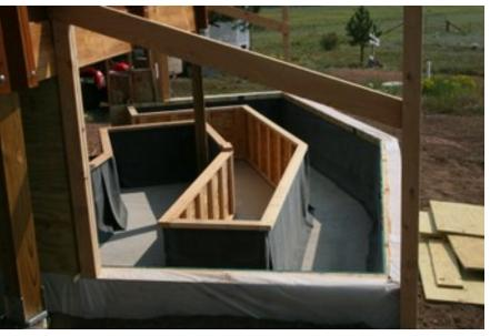
I also put spacers under the bottom plate to raise the plate off the concrete and to make it easier for any water to seep out and not just sit there and soak the plates for long periods of time. I used scrap pieces of the 3/4" PT plywood from the outside walls for this.
