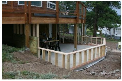
All the walls are 2x6 and are insulated with fiberglass batt insulation. I used 3/4" pressure treated plywood on the outsides of the walls. I got the kind that is rated for ground contact.
