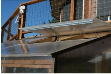
There are several models of this type of vent which vary in support load and cost. I went for the heaviest one mainly because I live in a high wind area and the return springs on a lighter model might not be able to withstand high winds. I also braced the vent from end to end with an L bracket.
