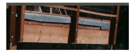
over the outside of the deck. This will lap on top of the GH roof when I build it. That will direct water that runs to the outside of the deck onto the GH roof where it will drain off.
