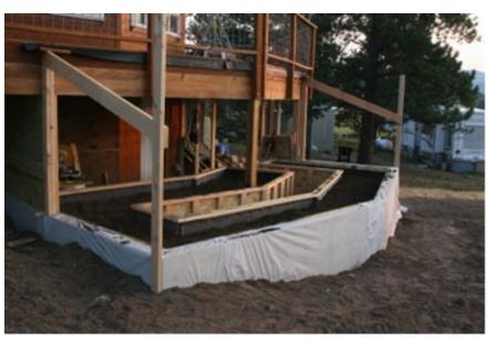
protection to the PT plywood. The outside walls will be covered with metal siding.
