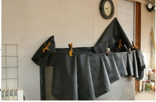
Note the angle iron running vertically on the left side of the sheet metal. I attached this to the wall running long screws all the way thru the wall and thru a flat piece of metal on the far side.
