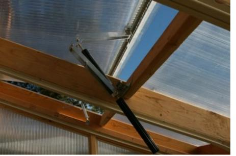
The piston is removed (unscrewed) at night when I need put up the insulation; it hangs below the rafters a bit.
