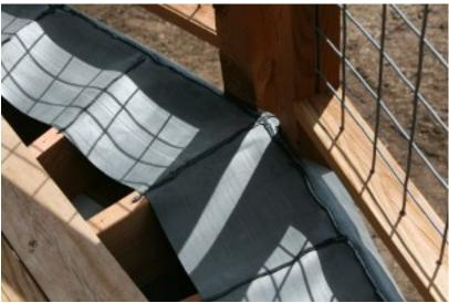
Water is captured by the EPDM and drained onto the sheet metal underneath, which is then dumped into the gutter.
